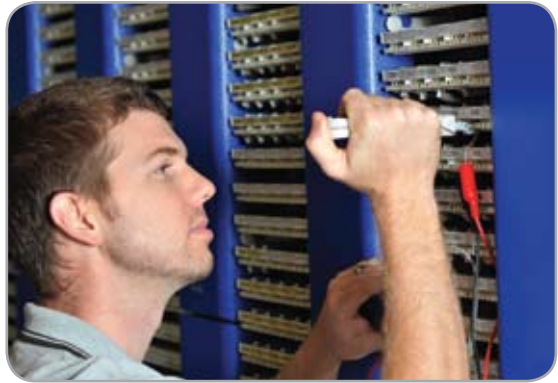
Patch-by-Exception termination with an ADC KRONE Sensor Tool
