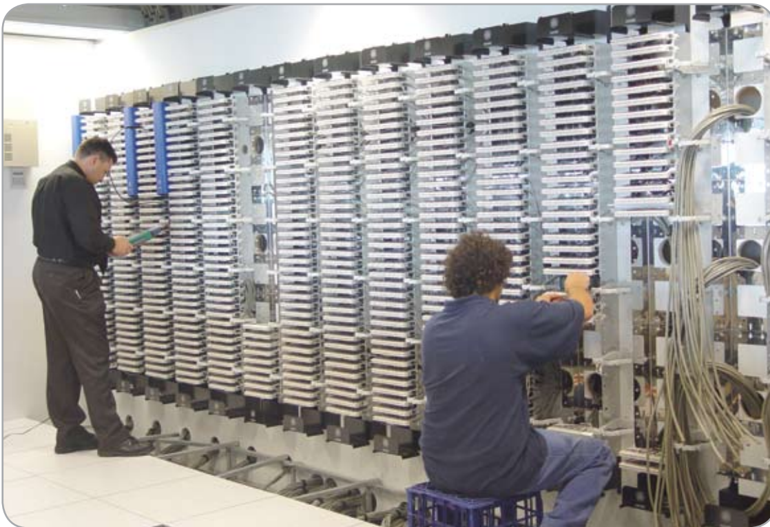
Tom Hammerl, Structured Communications and Alex Price, ADC KRONE, conduct permanent link testing.
