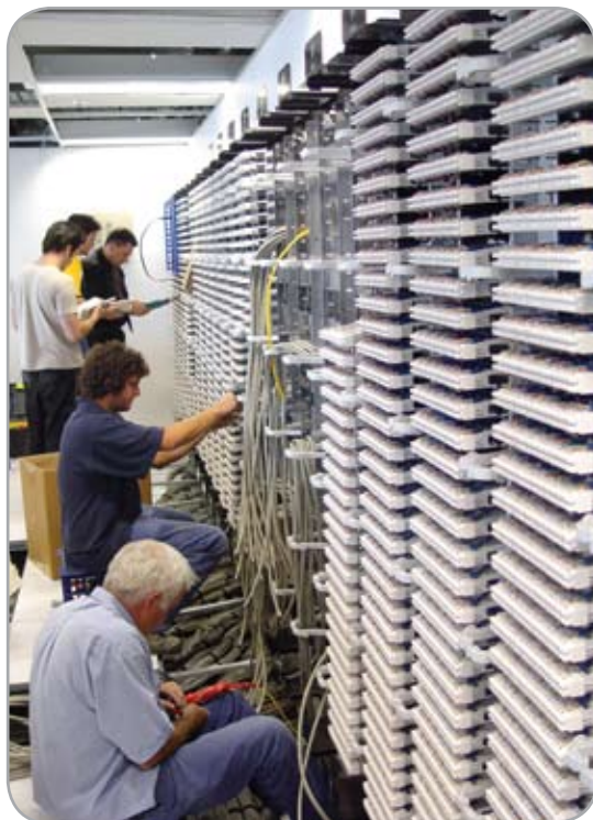
The team from Structured Communications terminate the HighBand 25 modules.
