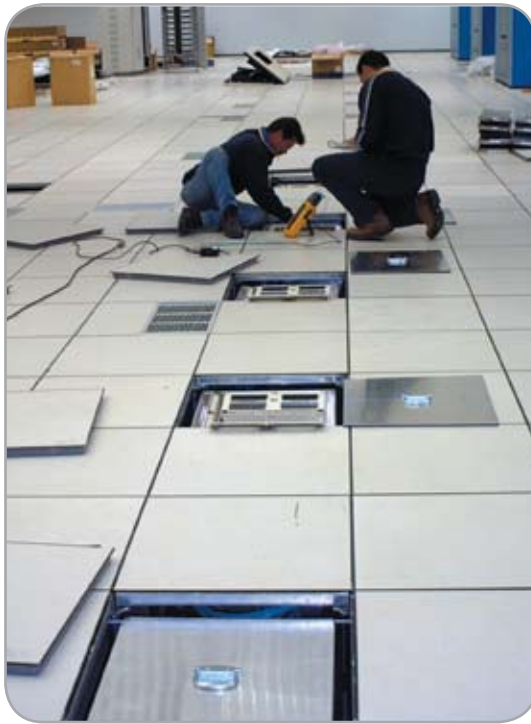
Technicians mount FL2000 fibre termination panels flush under the raised floor, providing interconnect access for adding, removing and rearranging servers.
