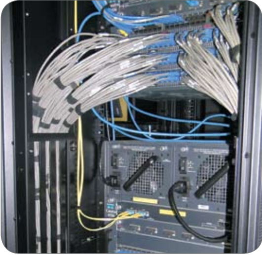
Patching into active equipment.
